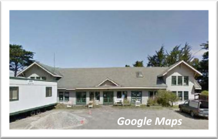
BCPUD Administrative Offices
