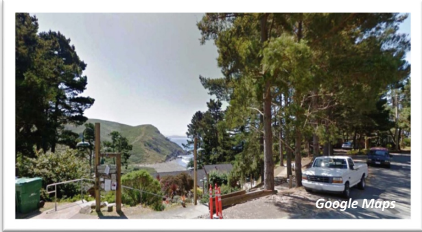
MBCSD Community Center
